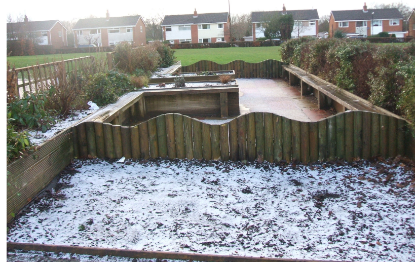
Supergrounds St Mary's RC Primary School
